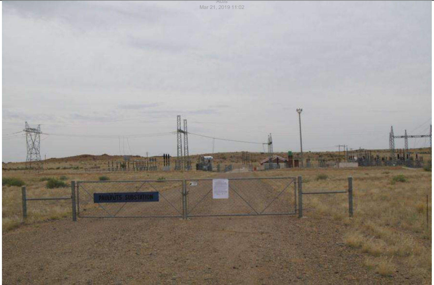
Site notice on Konkoonsies site boundary fence at Paulputs substation
