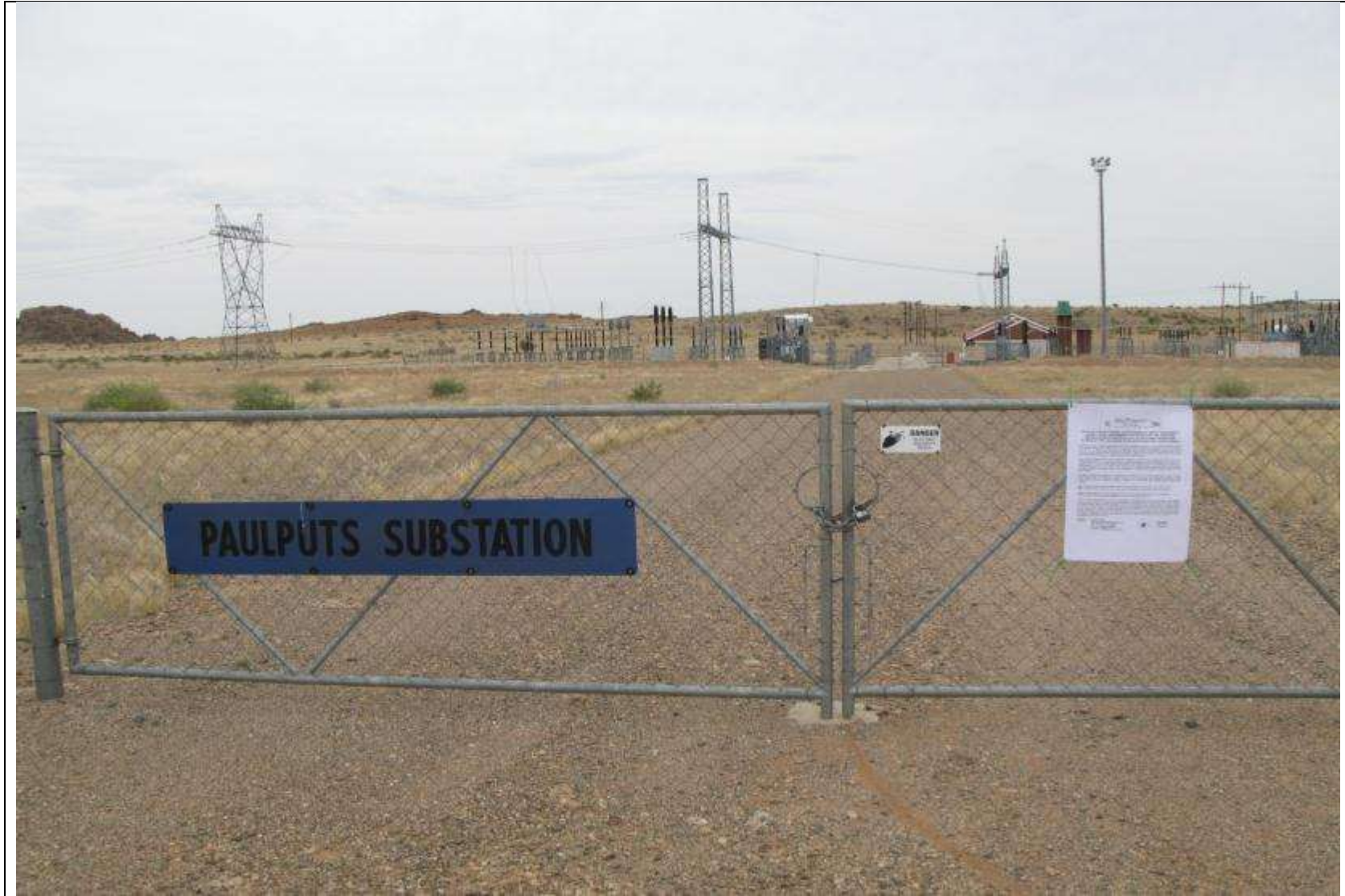
Site notice on Konkoonsies site boundary fence Paulputs substation
